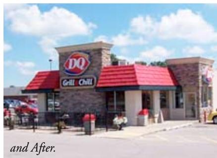
*Dairy Queen stores share standardized architectural features; for these projects The Hamstra Group is in charge of new exterior finishes, including stonework on chimneys and aluminum composite panels. Inside, floors and walls are ceramic tile and slate. This Demotte, Indiana, DQ is owned by Ted and Marybeth Vinyard.*
