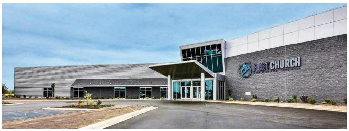
First Reformed Church utilized traditional steel framing with charcoal split-faced block. Silver aluminum composite panels and horizontal metal siding complete the look. The tilted windows over the entry doors, as well as the tilted wall in the front of the church, break up the look of the building and add visual interest. The two unique tapered and tilted entry canopies give the church a modern look.
