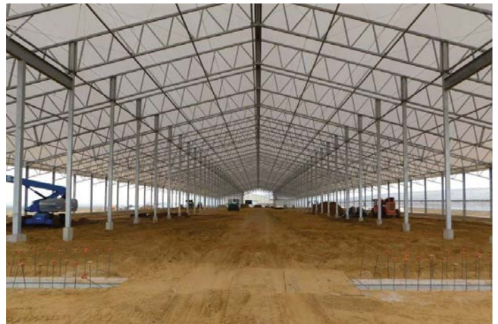
Pictured left: The bio-secure visitor center allows the public to visually participate in all aspects of the cows' routine—from eating and resting, to entering the milk production area. Right: During construction, we truly began to understand the scope of the project once the pre-engineered metal canopy was erected. Lots of space makes for happy cows!
