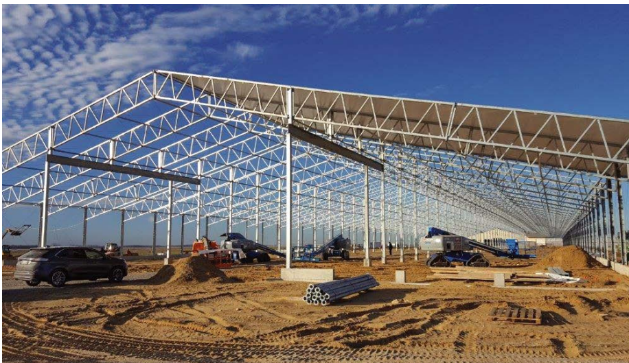
This $4.5 million design-build project was completed in just eight months.
